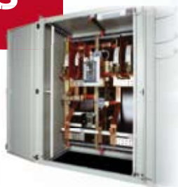
Sub-station electrical cabinet
